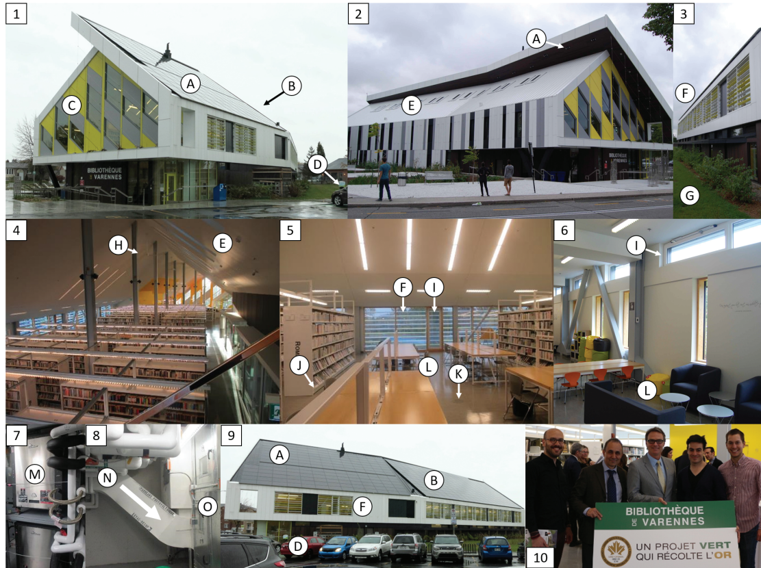
Figure 1 Varennes Library tagged images. (1) entrance, southwest view; (2) north façade; (3) south façade; (4) second floor, facing west, (5) second floor, middle section, facing south; (6) ground floor facing south; (7–8) mechanical room; (9) south façade; (10) official opening ceremony, from left to right: Dr. Konstantinos (Costa) Kapsis, Dr. Andreas K. Athienitis, Major Martin Damphousse, Vasken Dermardiros, and Remi Dumoulin. (A) forced convected BIPV and BIPV/T area; (B) naturally convected BIPV portion (out of view); (C) west façade, vine supports; (D) two car charging station; (E) skylights on northern roof; (F) fixed exterior louvers, solar shading; (G) geothermal boreholes; (H) ceiling fans; (I) motorized windows; (J) displacement ventilation integrated to bookshelves/stacks; (K) underfloor ventilation diffuser; (L) hydronic radiant slab; (M) geothermal heat pumps; (N) BIPV/T heat into air-handling unit (AHU); (O) AHU.
