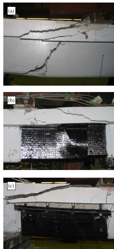
Fig. 6. Cracking and failure pattern of beams: (a) S-C-O; (b) S-E-B; and (c) S-M-D
