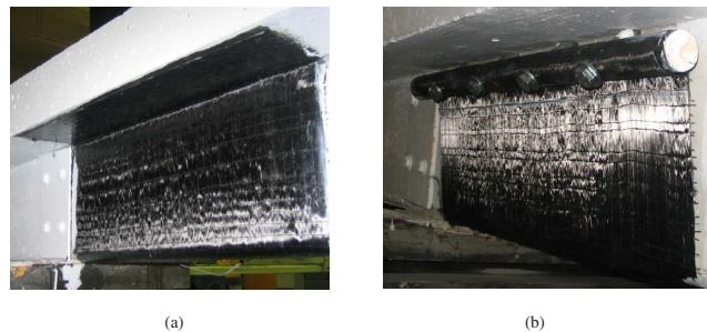
Fig. 4. Detailed view of the strengthened beams before test: (a) S-E-B; (b) S-M-D
