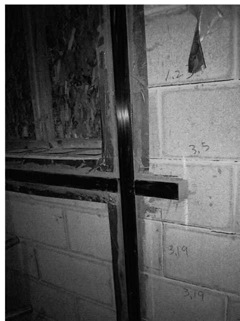
Fig. 2. Carbon fiber-reinforced polymer strips before removing the duct tape
