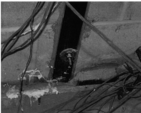
Fig. 4. Carbon strip anchored at bottom of wall
