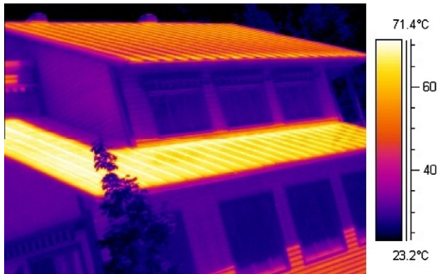
Fig. 5. Thermographic image of BIPV/T roof (upper roof section) compared with the lower metal roof section.
