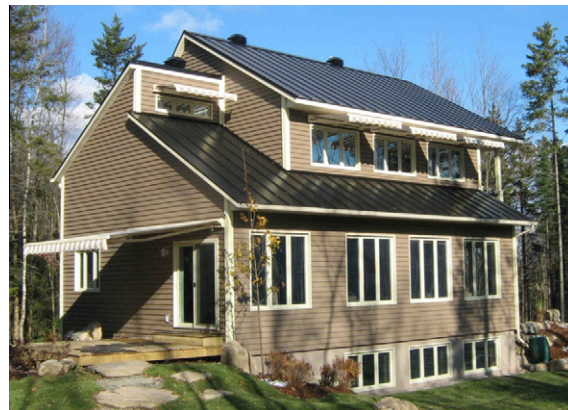
Fig. 1. ÉcoTerra demonstration house, November 2007 (the photovoltaic system made up of amorphous laminate panels attached to metal roof is on the upper roof section).
