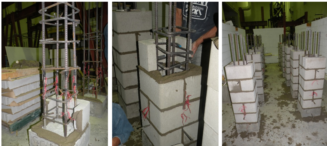
Fig. 4. Construction sequence of placing steel bars and blocks in the C-RMBEs.
