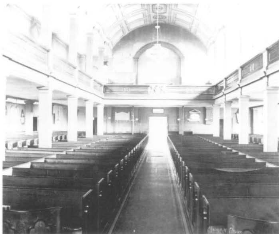
fig.15 St. Paul's Church, interior, view to north, ca. 1891, photograph by William Notman Studio. Coll.: PANS. (Photo: courtesy PANS.)
