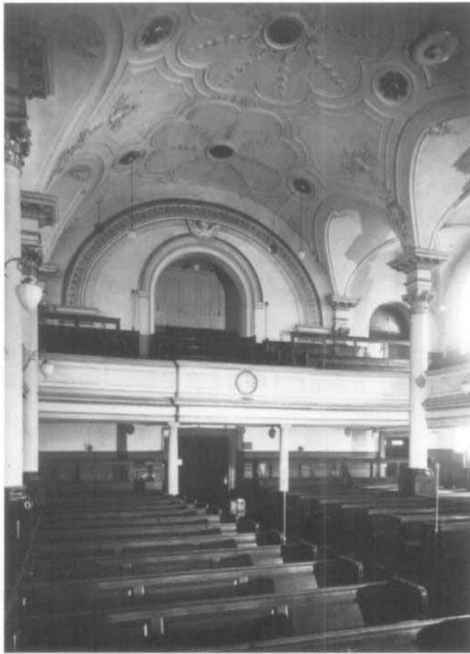
fig.10 St.Peter's, Vere Street, interior, view to west. (Photo: courtesy National Monuments Record, London.)
