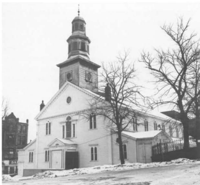
fig.1 St.Paul's Church, Halifax, exterior, view from north, 1970.
