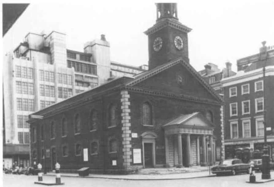
fig.5 James Gibbs, St.Peter's, Vere Street, London, 1721-24, exterior, view from northwest. (Photo: courtesy Courtauld Institute of Art, London.)
