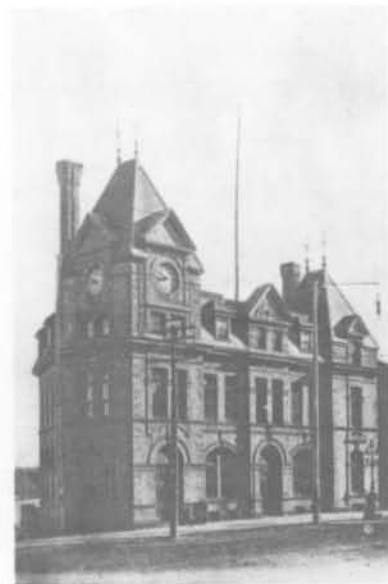
Fig. 3. T. S. Scott, Post Office, Customs and Inland Revenue Building, north side of Ontario St., Stratford Ont. Designed in or before Sept. 1881. Contract signed 16 January 1882. (Photo: before 1894, Perth County Archives).
