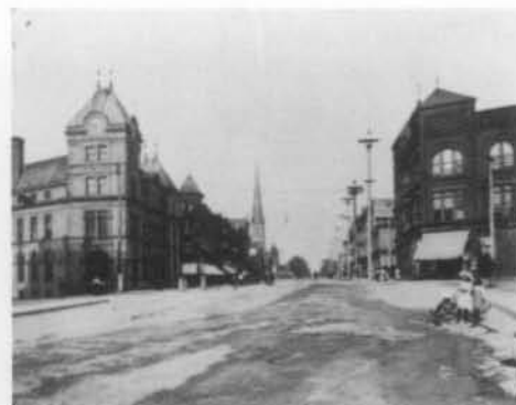
Fig. 7. Stratford Ont. Ontario Street looking east from a point just west of Erie St.: Post Office (left), Gordon Block, 1902 now threatened (right), tower of Knox Presbyterian Church, distance (burned). (Photo: Perth County Archives).
