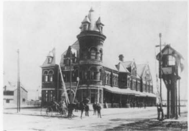
Fig. 26. TH&B Railway Station, Hamilton. (Photo: Ontario Archives).
