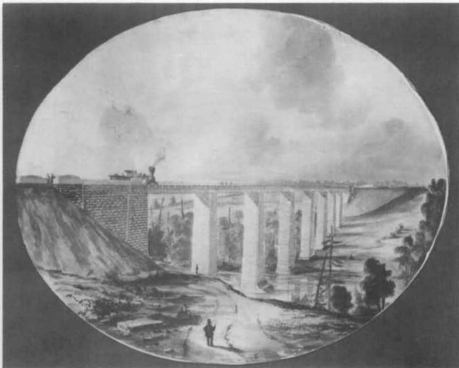
Fig. 18 GTR Viaduct, Georgetown, Ont. (Photo: Royal Ontario Museum).
