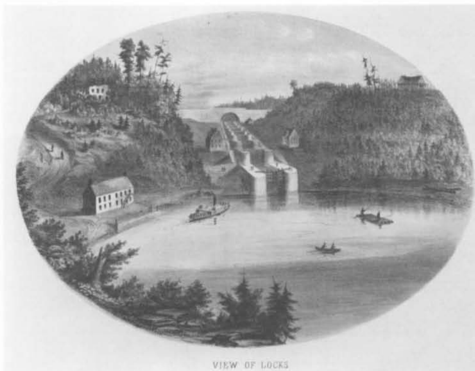
Fig. 5. The first Eight Locks on the Rideau Canal, Ottawa. (Photo: Royal Ontario Museum).
