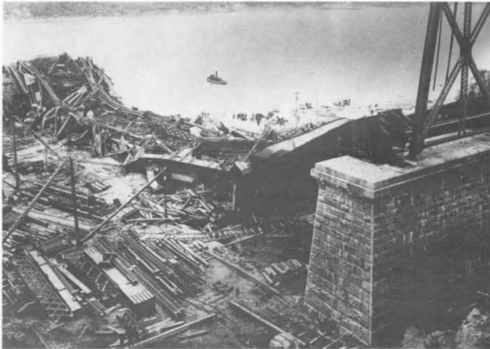
Fig. 16. The collapse of the Quebec Bridge while under construction. (Photo: National Museum of History & Technology, Smithsonian Institution).
