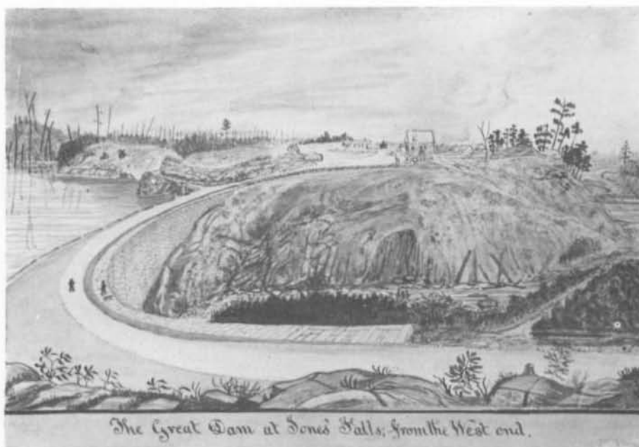
Fig. 6. The Jones Falls Dam on the Rideau Canal. (Photo: Ontario Archives).
