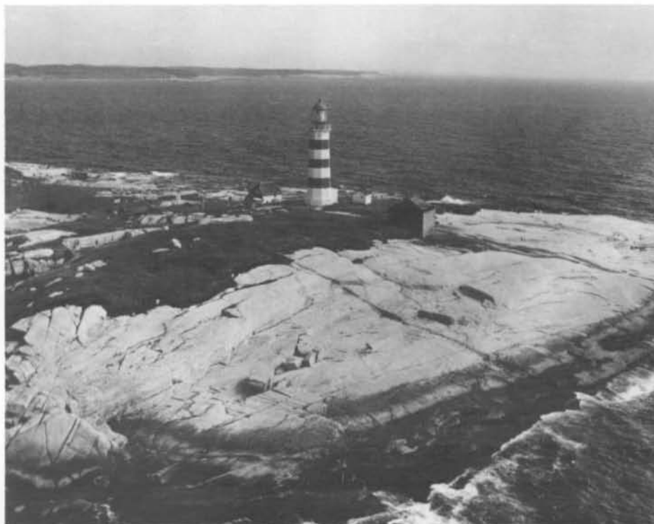
Fig. 1. Lighthouse, Sambro Island, N.S. (Photo: Nova Scotia Communication & Information Centre).
