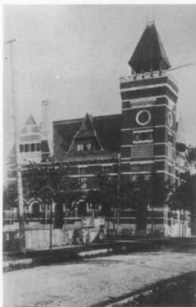
Fig. 22. Thomas Fuller, Customs and Inland Revenue Building, corner Queen and Hector Sts., Port Hope Ont., cornerstone laid 30 August 1883. (Photo: Province of Ontario Archives).
