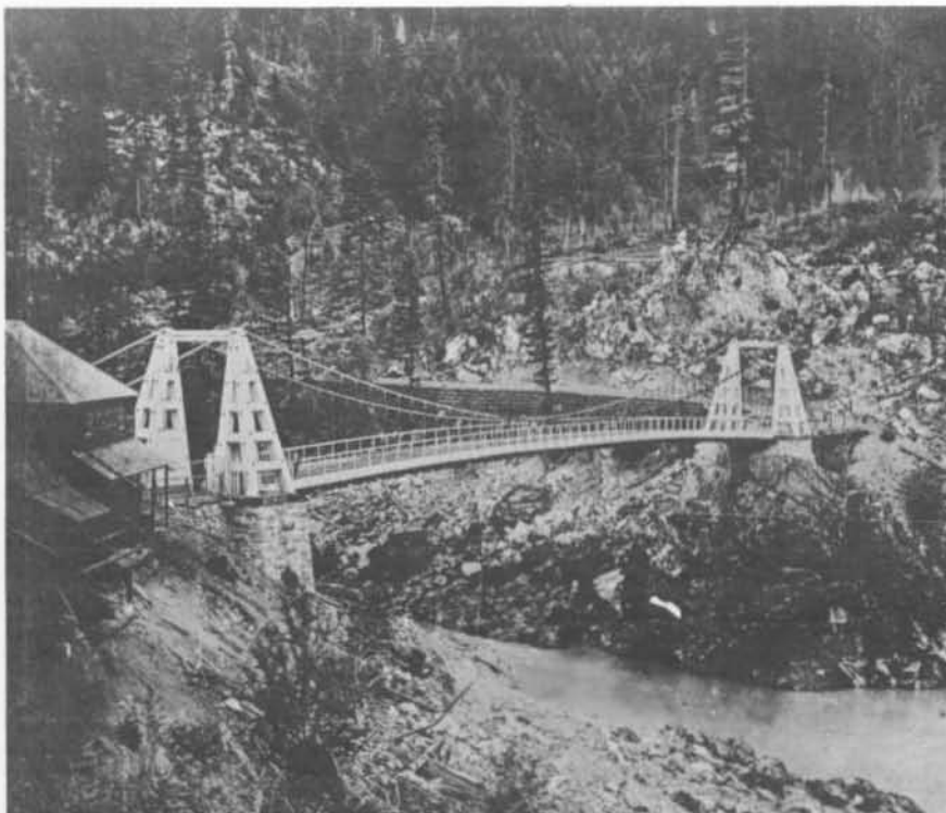
Fig. 11. The Alexandra Suspension Bridge and the Cariboo Wagon Road at Spuzzum, B.C. (Photo: Archives of British Columbia).
