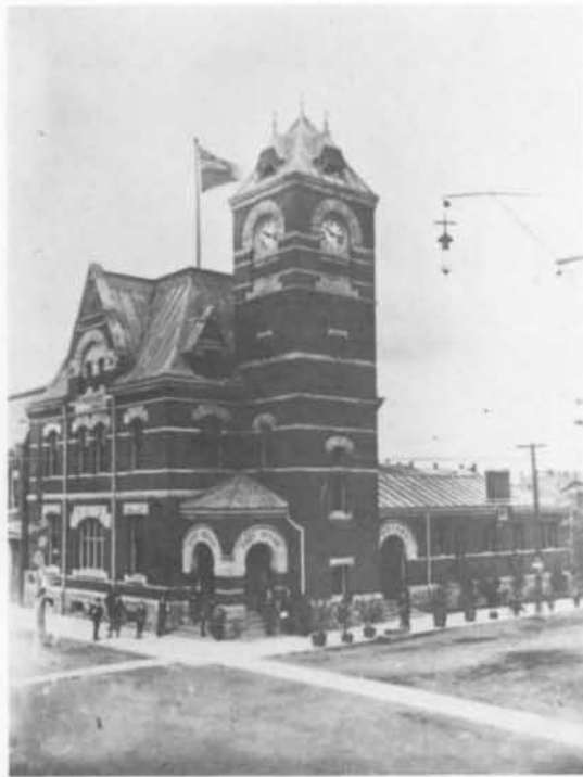
Fig. 1. Thomas Fuller, Post Office, Customs and Inland Revenue Building, corner Frank and Centre Streets, Strathroy, Ont. Contract signed 31 July 1889. (Photo: The Age-Dispatch ).
