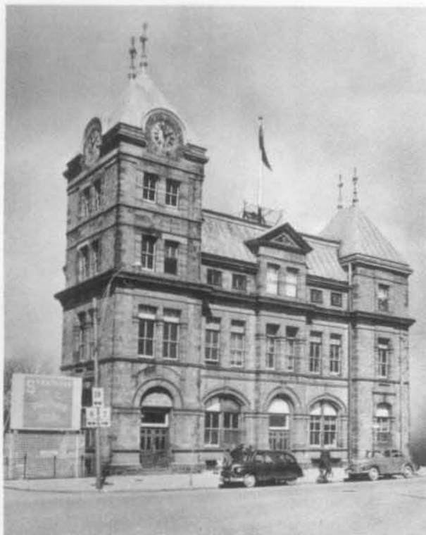
Fig. 6. T. S. Scott, Post Office, Customs and Inland Revenue Building, Stratford Ont. Shortly before demolition in 1961. (Photo: Stratford Beacon-Herald).
