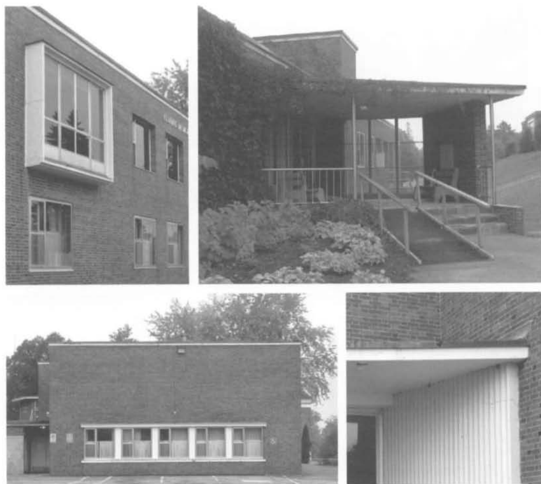
fig. 5 UNB Memorial Student Centre exterior features, clockwise from top left: precast concrete window surround; angled rear entry porch; horizontal ribbon of aluminum windows at side elevation; and fluted concrete decoration at front entrance. (Photos: the author)
