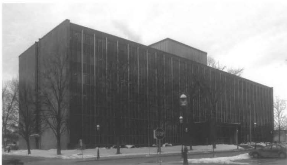
fig.12 Centennial Building, Fredericton, NB, completed 1967. Architect: Bélanger & Roy. (Photo: the author)
