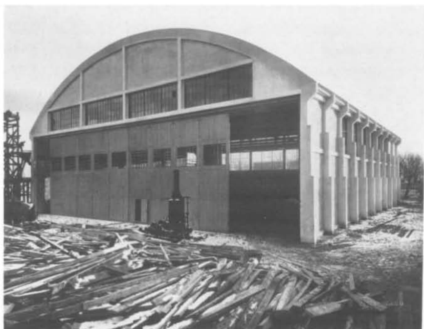
fig. 14 Ernest Cormier, architect, Hydroplane Hangar, Airport, Pointe-aux-Trembles, 1928, 19.1 × 24.2 m, Montréal, Collection Centre Canadien d'Architecture / Canadian Centre for Architecture, AR01:P-1804. (Photo: anonymous photographer, 1930)
