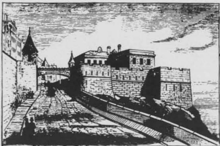
MOUNTAIN HILL.—Iron Bridge.
