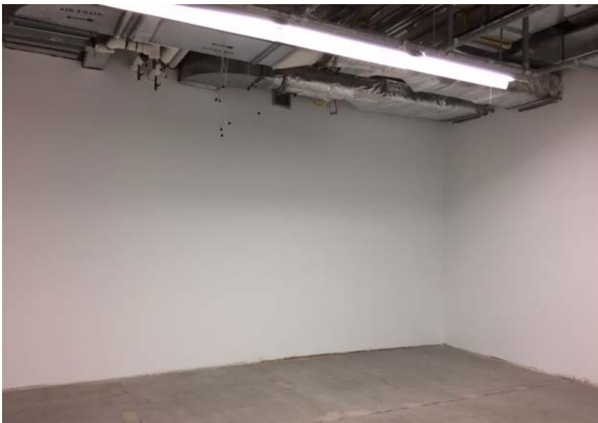
EV4.525 Photo Grad Space
