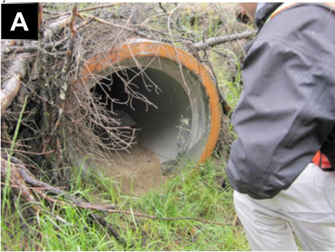
Round concrete culverts, can have a diameter of either 60 cm or 90 cm.
