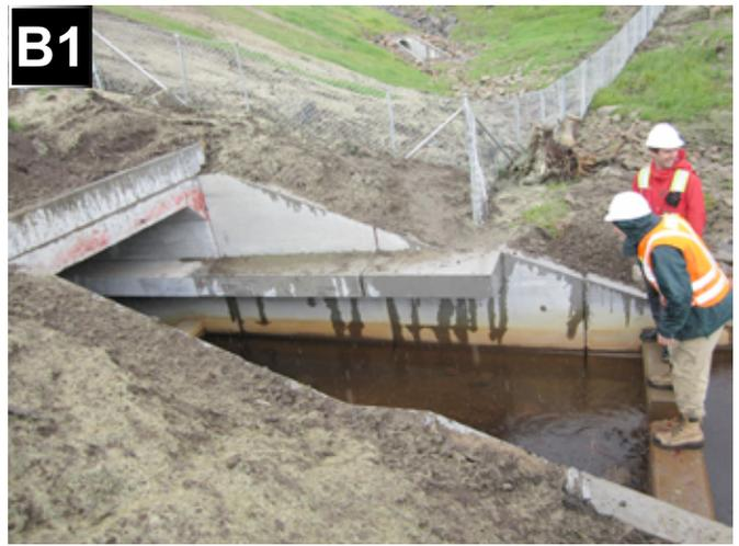
Box culverts with a prefabricated shelf in concrete.
