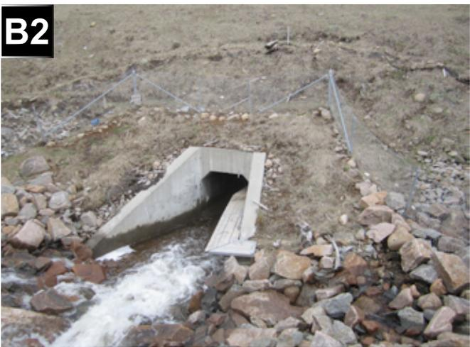
Box culverts with a wooden shelf built on as an addition.
