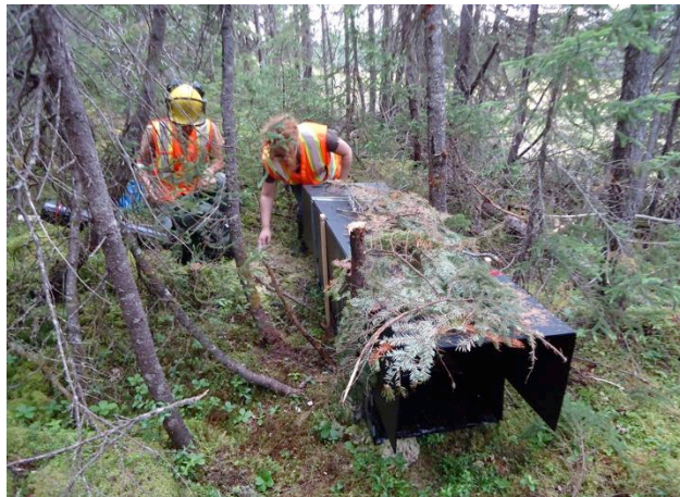
Figure 8: Track box being installed in the forest.
