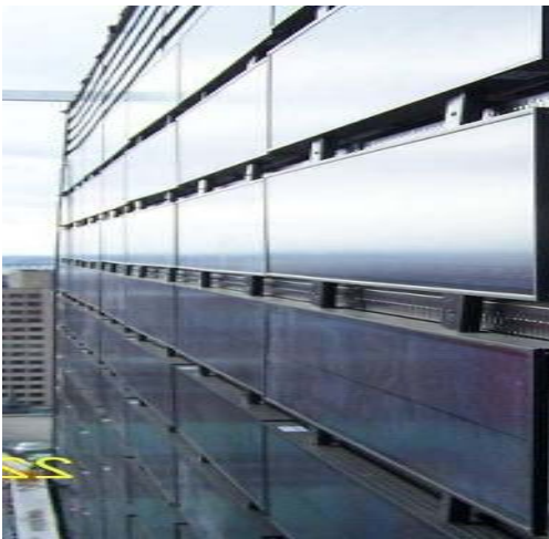
Close-up view of PV panels over UTC* cladding
