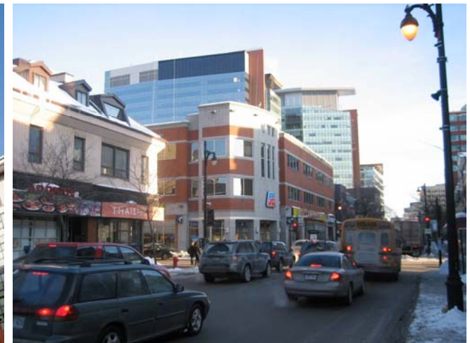
BIPV/T system seen during JMSB building construction from downtown Montreal
