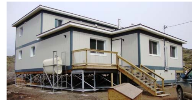
Arctic house with hot roof design changed to an unventilated cold roof, Iqaluit, Nunavut.
