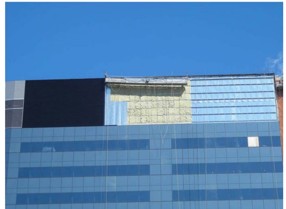
System with a finished portion of UTC, thermal insulation and metal sheathing
