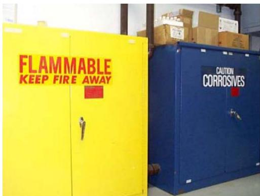
Figure 8. Specific types of storage cabinets must be specified in laboratories in order to separate incompatible chemicals from one another and to safely store all chemicals.
