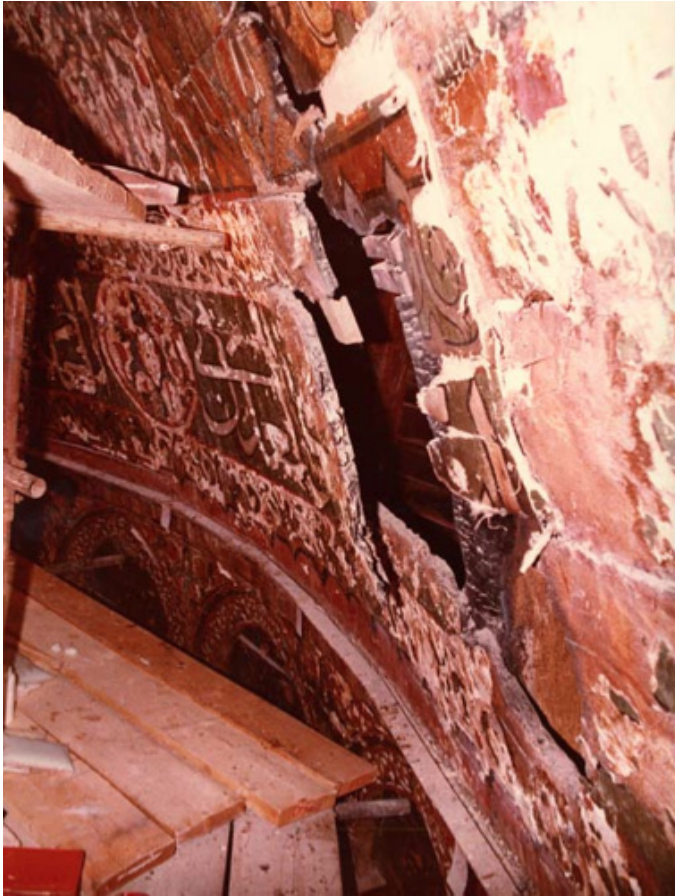
Fig. 4. Isam Awwad, Interior Fire Damage to the Interior Dome of al-Aqsa Mosque. Photograph, 1983. Al-Aqsa Mosque, Al-Haram al-Sharif, Jerusalem. Courtesy the Aga Khan Award for Architecture.
