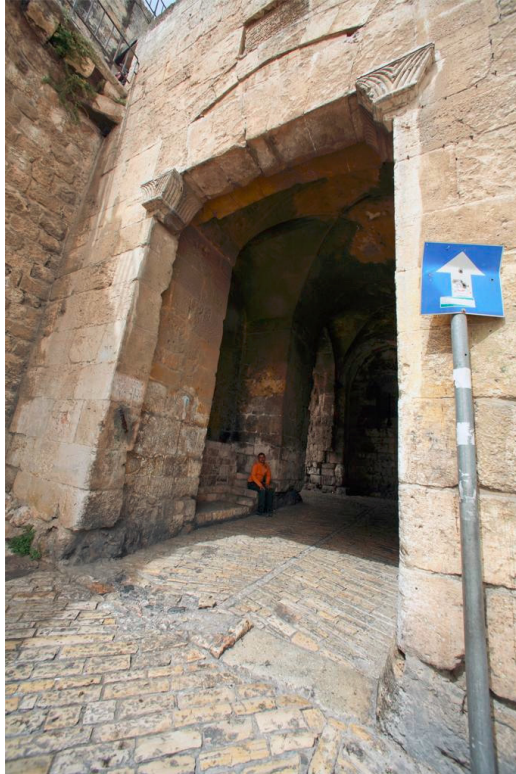
Fig. 4. Zion Gate. View of north façade. Jerusalem.
