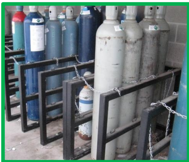
Figure 11.2.1: Proper and improper ways to store gas cylinders. (ref: waltbeattie.com; en.wikipedia.org)
