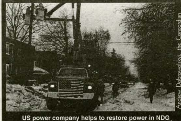
US power company helps to restore power in NDG.
