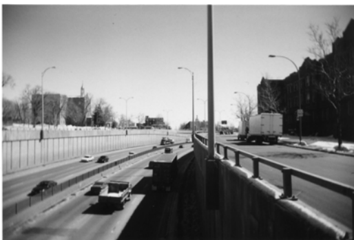
Figure 2.1 Décarie Autoroute; a scar in the urban fabric of Notre-Dame-de-Grâce
