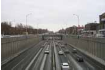
Figure 2.3 Décarie Highway, facing South.
