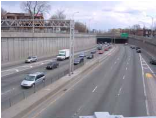
Figure 3.11 Facing South West on Décarie Boulevard
