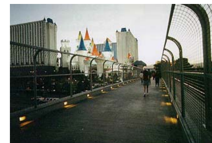
FOOT BRIDGE B
