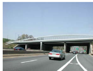
FOOT BRIDGE A
