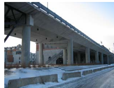
BRIDGE FACING WEST
